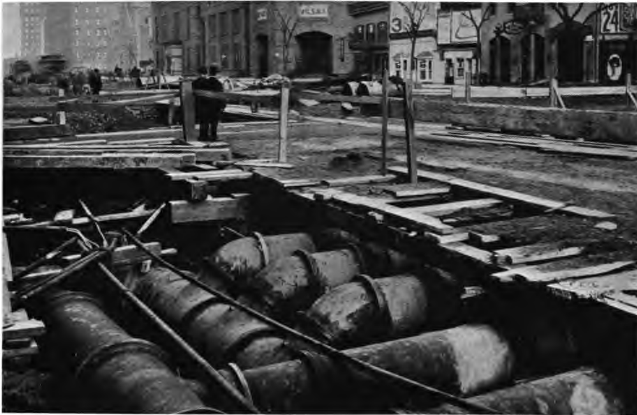
SUBDIVISION OF 36" AND 30" GAS MAINS OVER ROOF OF SUBWAY—66TH STREET AND BROADWAY
